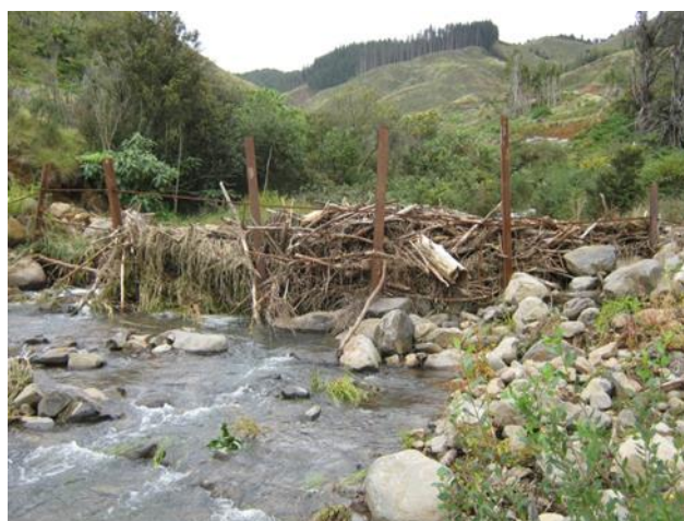
Figure 16: Photo of a slash trap.
